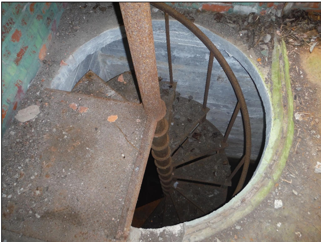
Figure 11. View of the Laurinburg Pump Station, staircase, facing northwest.
