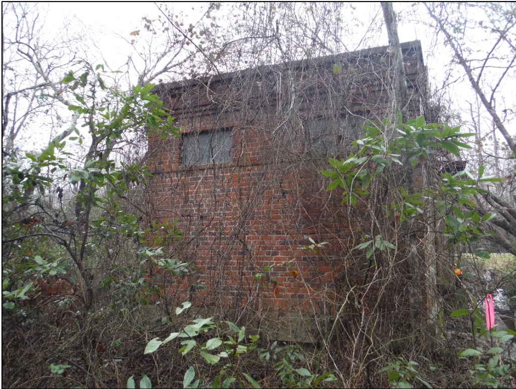
Figure 6. View of the Laurinburg Pump Station, facing northwest.
