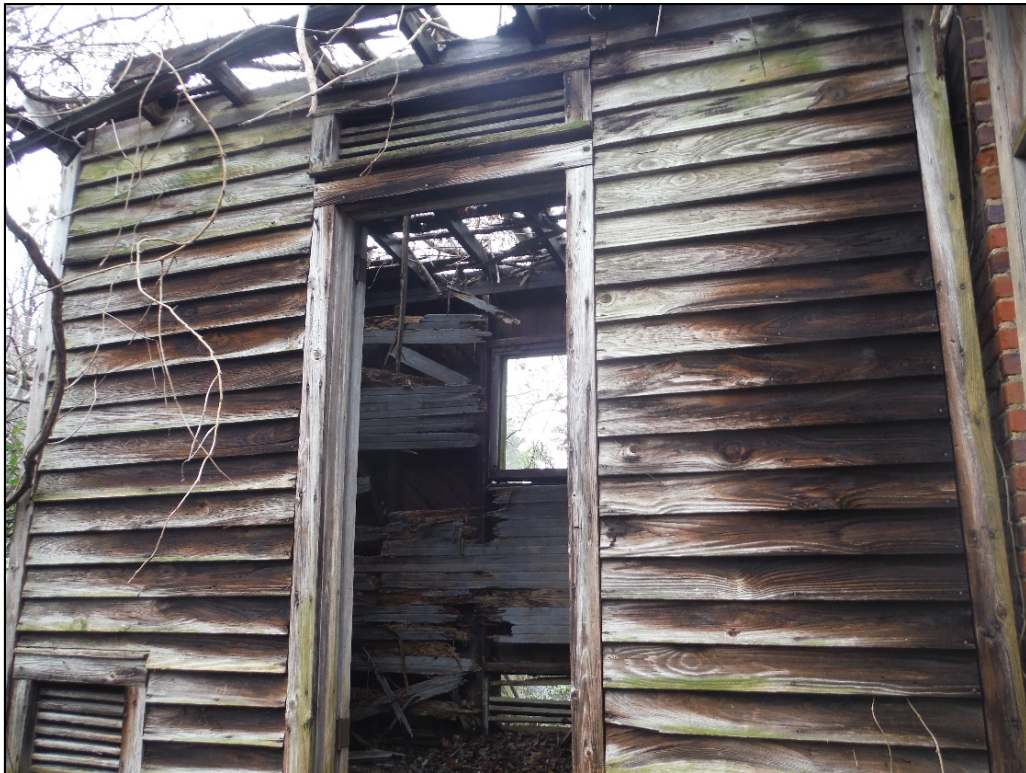
Figure 10. View of the Laurinburg Pump Station, wooden extension, facing north.
