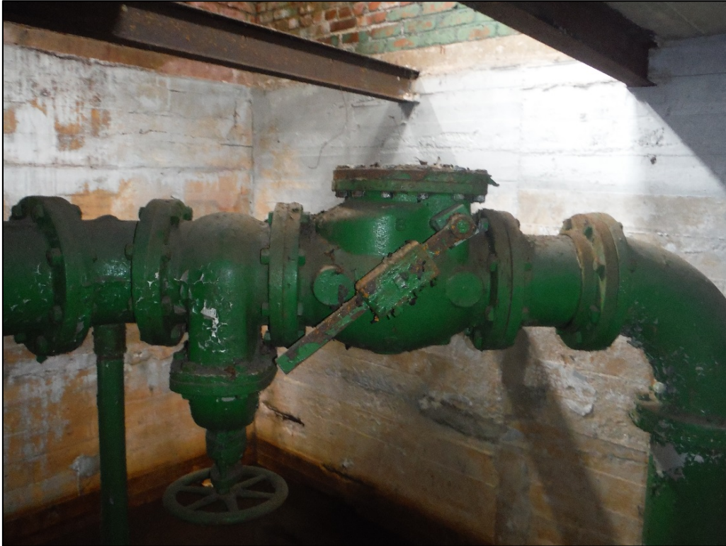
Figure 12. View of the Laurinburg Pump Station, pipes, lower story.
