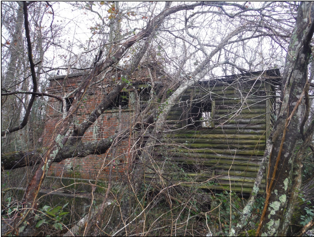
Figure 3. View of the Laurinburg Pump Station, facing southeast.
