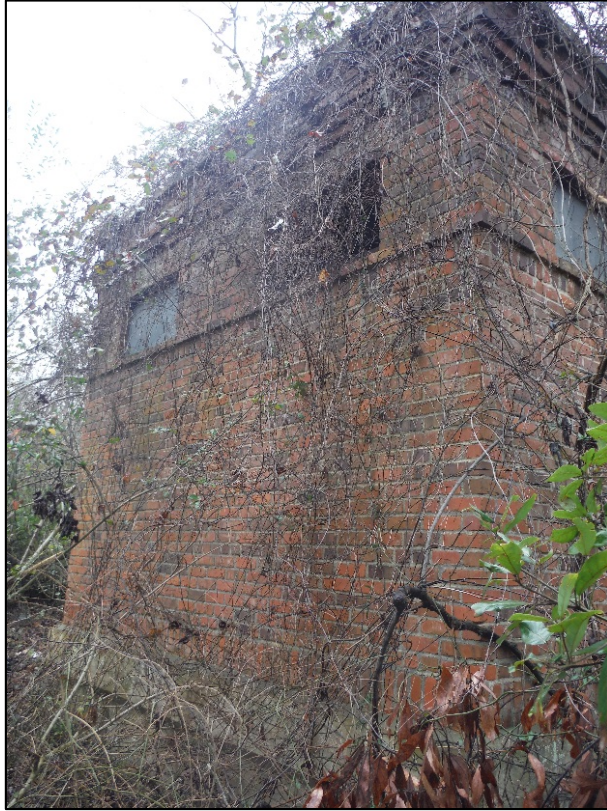
Figure 7. View of the Laurinburg Pump Station, facing north.
