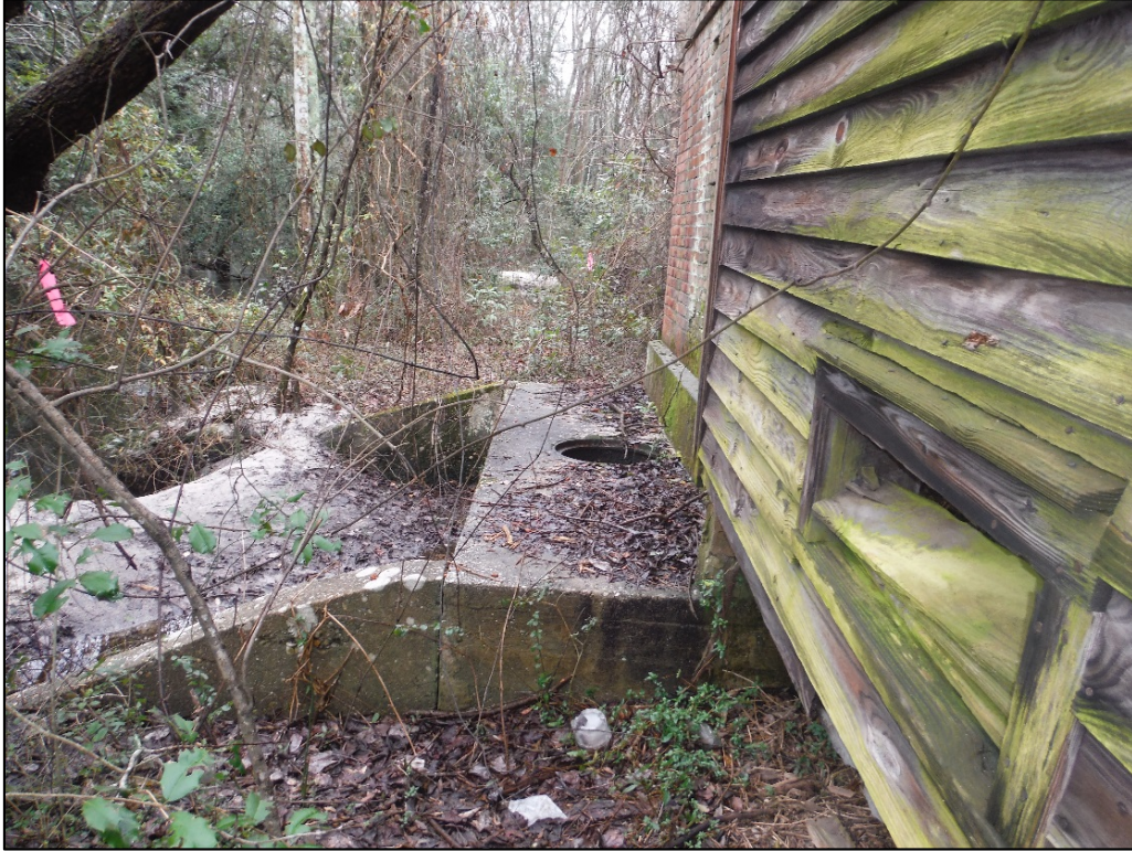
Figure 16. View of the Laurinburg Pump Station, drain, facing southeast.
