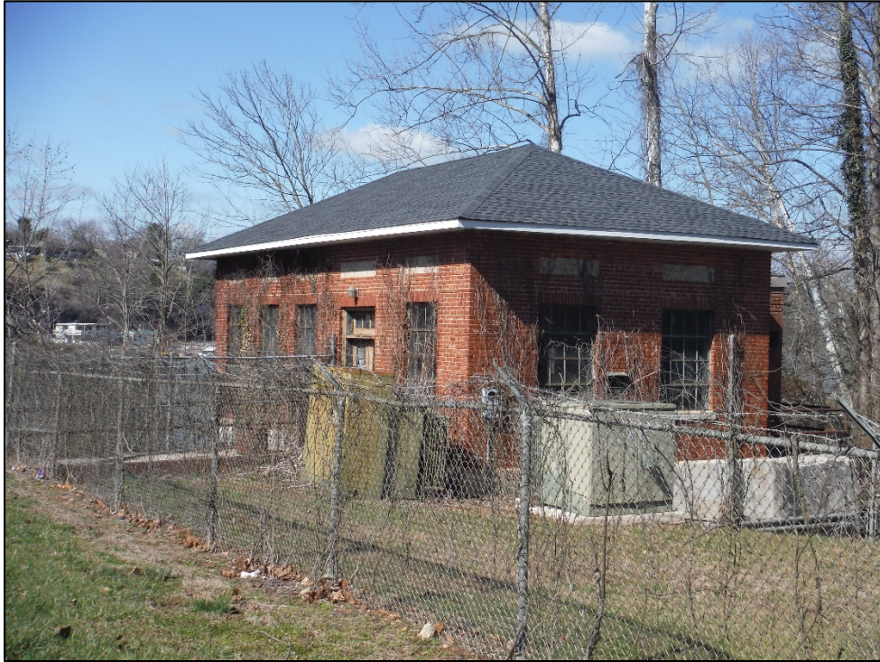
Figure A1. View of the Hickory Waterworks Pumping Station (BK0362), facing north.
