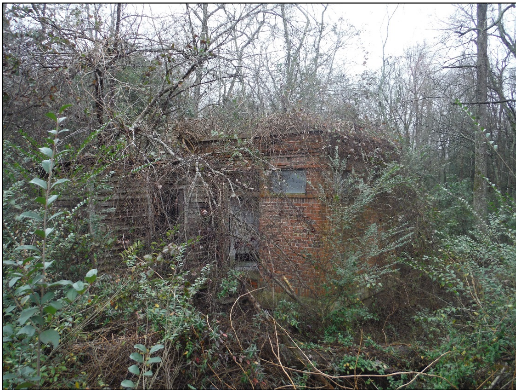
Figure 8. View of the Laurinburg Pump Station, facing east.
