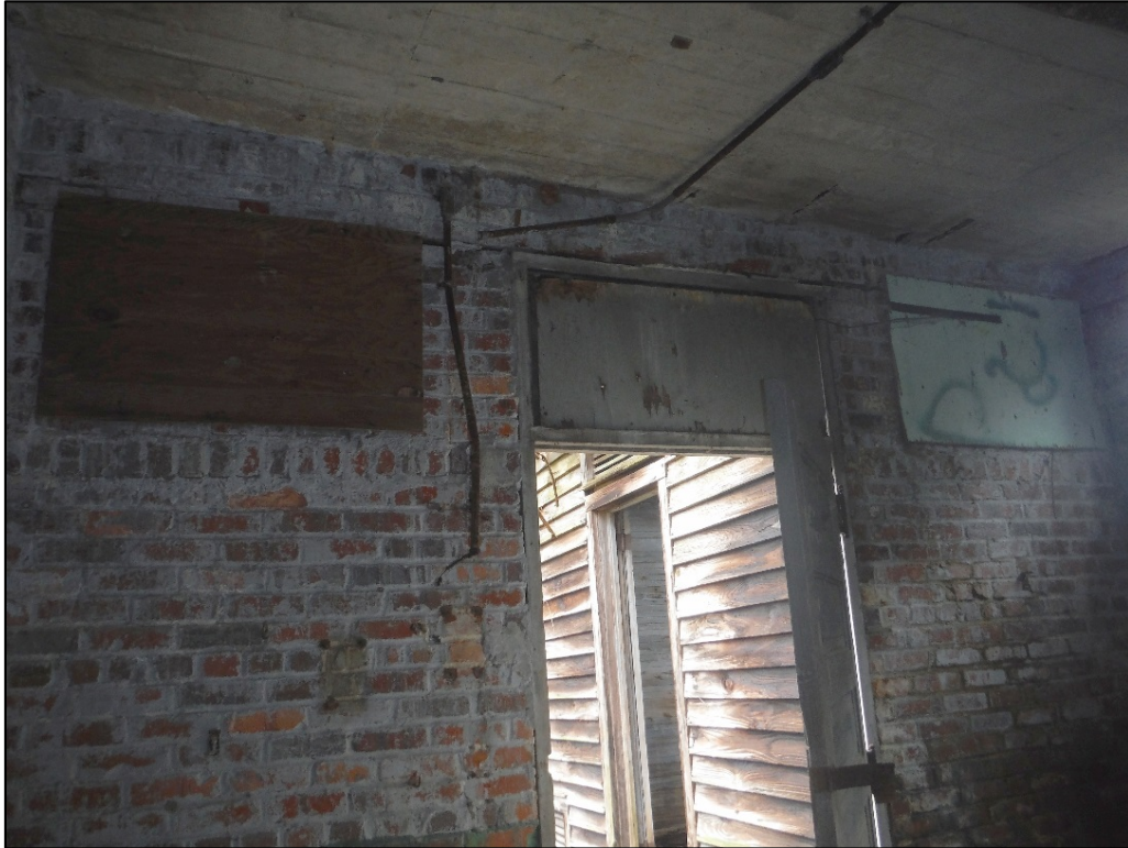
Figure 14. View of the Laurinburg Pump Station, interior facing northwest.
