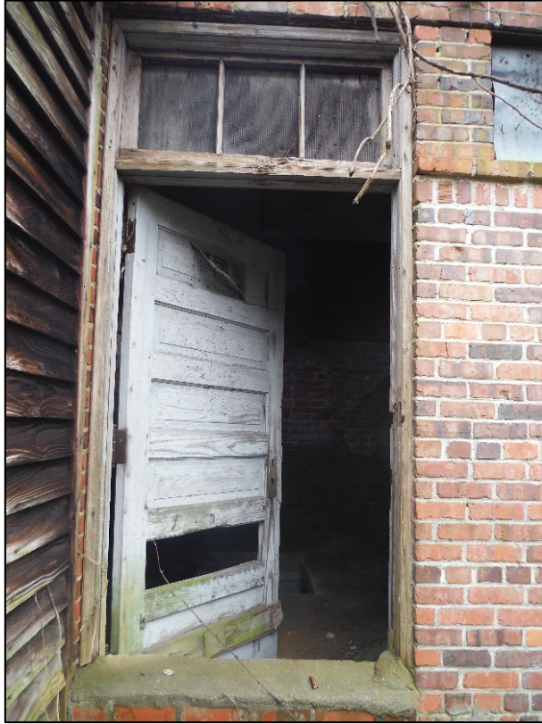
Figure 9. View of the Laurinburg Pump Station, entry detail, facing west.
